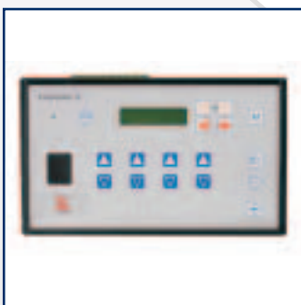
Detail of O 2 control, installed on the front of the panel
